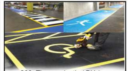
209. Thermoplastic / PU / Epoxy Marking
